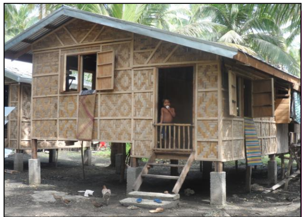
One of the 35 core shelter units constructed under the ERRCM Project
