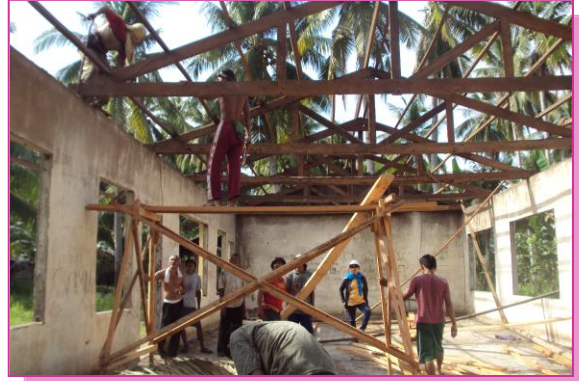
MWDECC totally renovated the school facility in Barangay Gawang.
