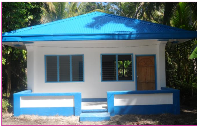
1 unit Barangay Health Station constructed in Barangay Gawang to help improve the access to and delivery of health services in the community
