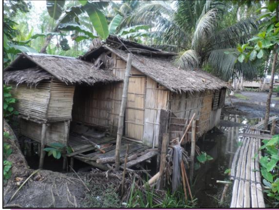
One of the houses in Barangay Gawang prior to the ERRCM Project
