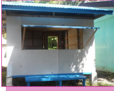
Botika ng Barangay (BnB) constructed in Barangay Gawang
