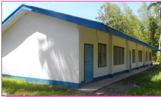
The newly renovated school facility provided with educational materials and equipment to ensure its operation
